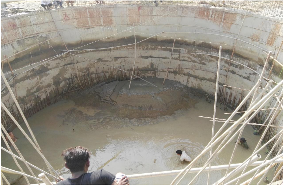
A view of Sump Well at WWTP during dewatering
