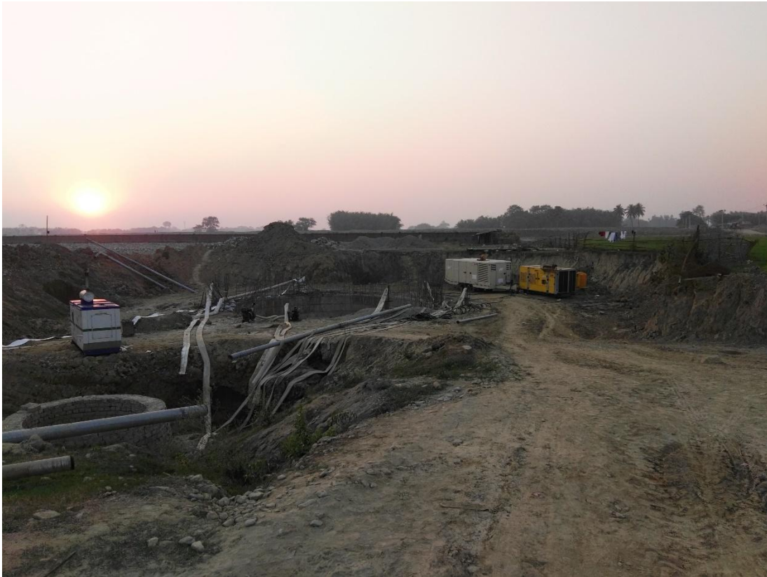
A view of Sump Well at WWTP – Preparation for dewatering
