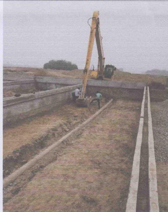
SDB filter preparation work
