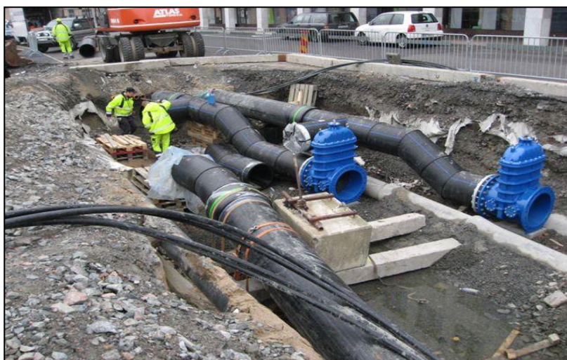
Construction of pre-insulated distribution pipes.
