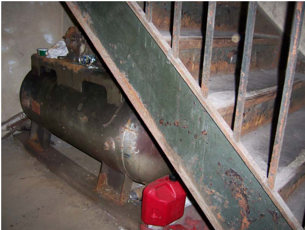
Photo 9: View of small AST located in the basement underneath the staircase in the south-southwestern portion of the building.
