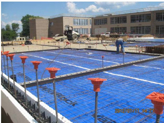
Concrete Slab On Grade – Preparation
