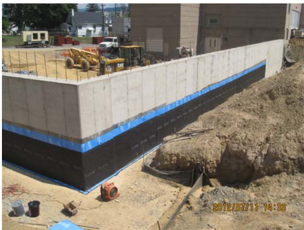
Area D –Mechanical Room Foundation Walls
