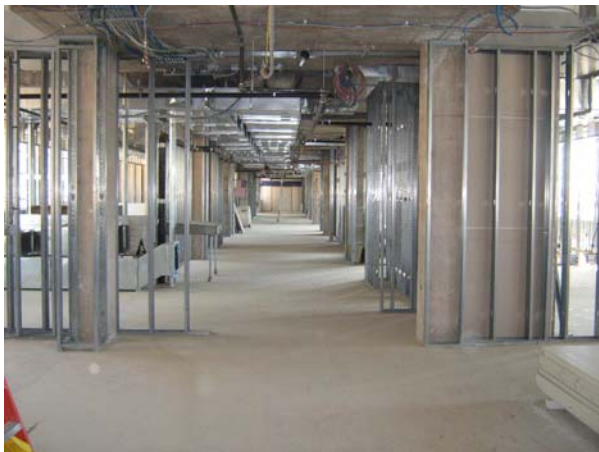
Metal Stud Wall Framing -2 nd Floor
