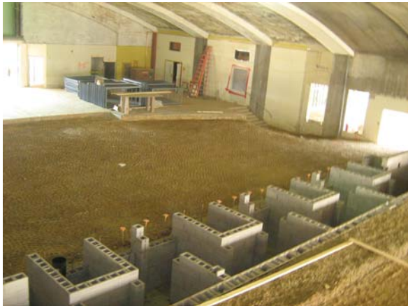
Cafetorium and Stage Area backfill
