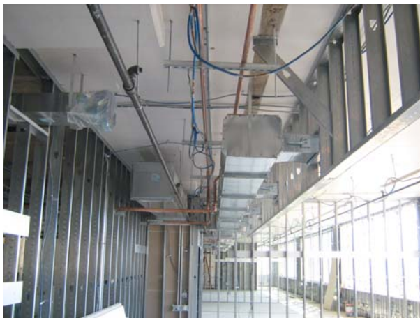
HVAC Duct Work Rough-ins
