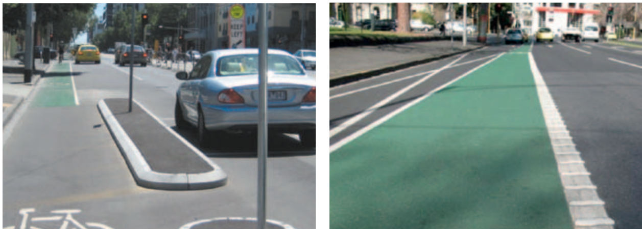
Figure 7 - Bicycle lane designs in the City of Melbourne. Physically-separated route Swanston Street (north) and green pavement and profiled edge-line treatments in Rathdowne Street
