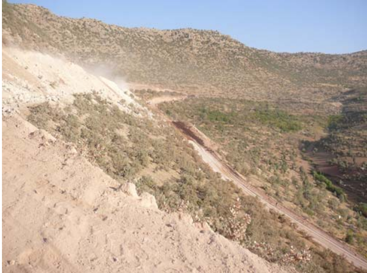
Photo 8: Road between Dargeçit and Ilisu construction site
