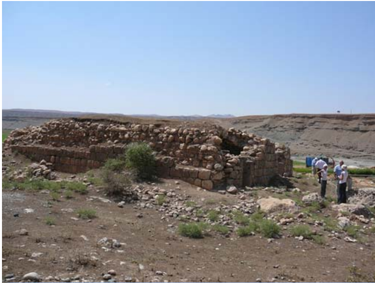
Photo 7: Post station of Sevgi Han (Botan valley)
