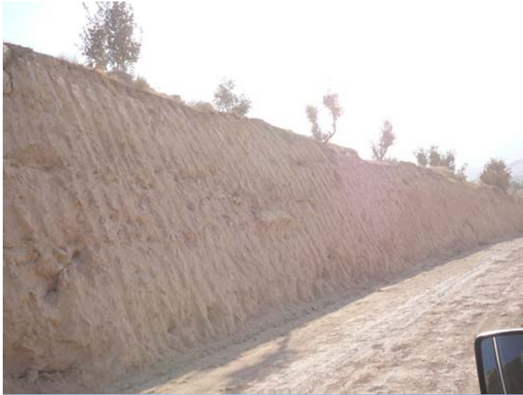
Photo 10: Enlargement of street near Ilisu construction site
